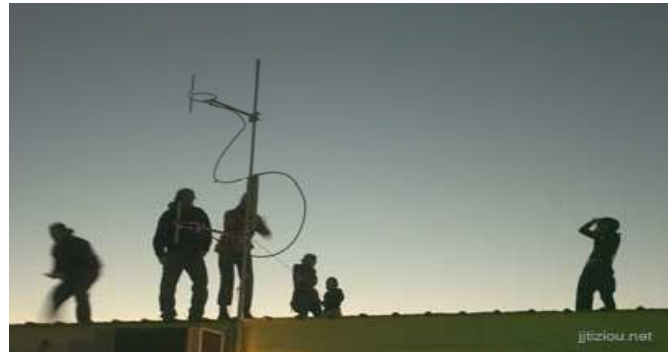
Volunteers raise the mast of WCIW-LP 107.9, Radio Consciencia, a station licensed to a farmworkers' group, the Coalition of Immokalee Workers, in Immokalee, FL.
