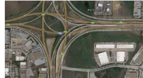
Goodrich Warehouse Built in 2007
