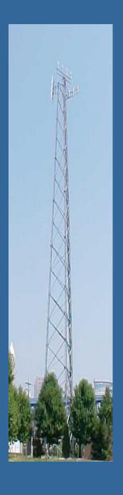
When the lighting change for an existing tower has been granted by the FCC via ASR, the steady-burning, side-marker, L-810 tower lights can be extinguished. This is typically accomplished in the tower transmission building and does not ordinarily require climbing the tower. For new towers, once the registration is granted, simply construct the tower without installing L-810 lights.
