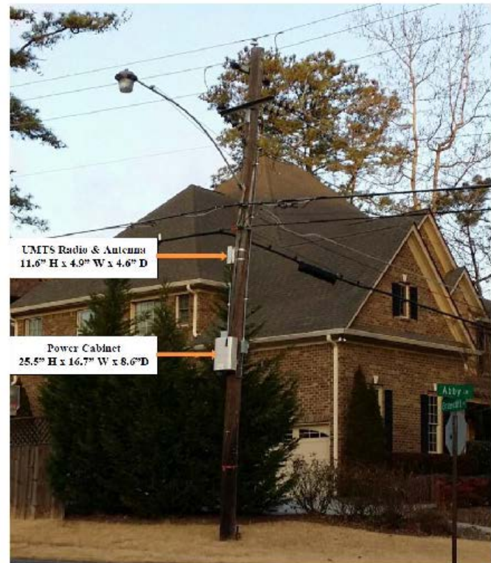
Pictures of Typical Small Cell and DAS Deployments
