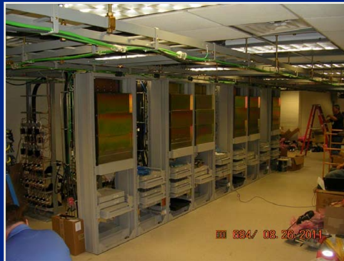
Carrier Base station equipment to connect to their macro network
