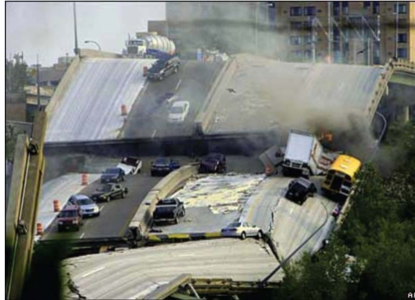
Figure 1 – Minneapolis Bridge After Collapse
